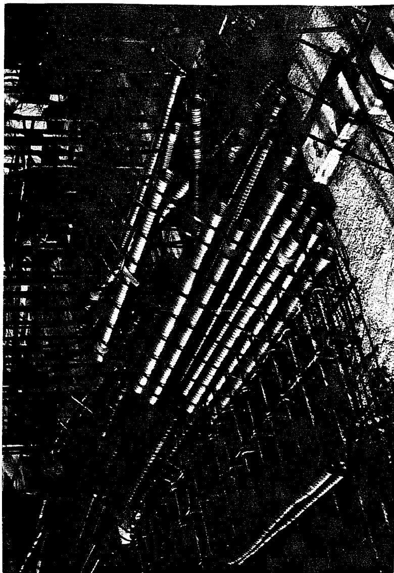
Figure 1.1 Congestion of Ducts for Internal Tendons
